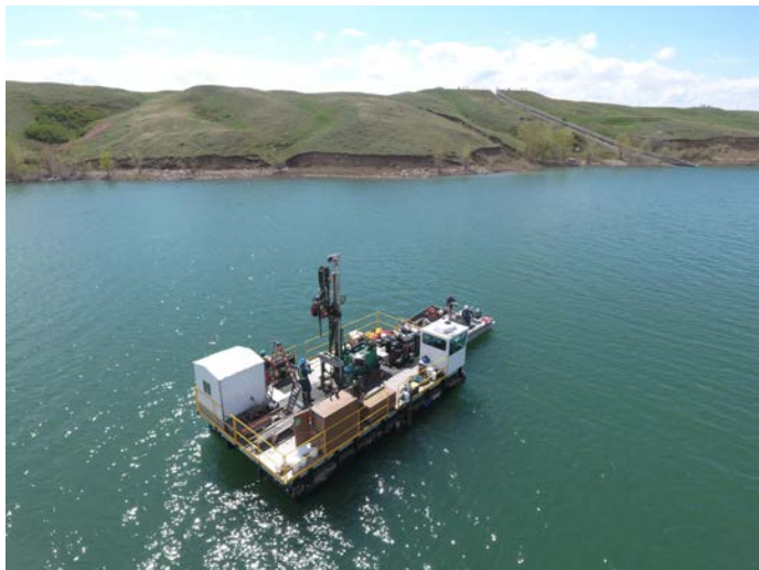
Fall 2023, Geotechnical investigation for planned refurbishment and raising of Chin West Dam. Amphibious drilling program
