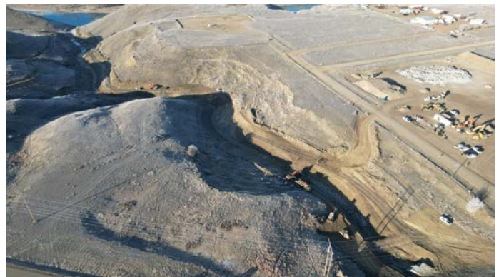
January 4, 2024 Drone photo of the 'Coulee' section of the spillway channel construction. DeGraaf Excavating was preparing the channel excavation for riprap and bedding material placement.
