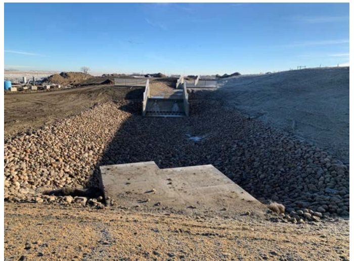
January 4, 2024 Looking east from Range Road 164A at the twin outlet of the 3 m x 3 m precast concrete box culvert in the foreground, which conveys water under Range Road 164A and two cast-in-place concrete drop structures in the background aligned along the spillway channel.
