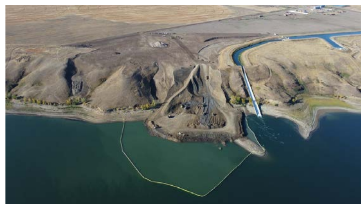
September 2023, Chin Chute Refurbishment Site Grading and Construction of cofferdam.
