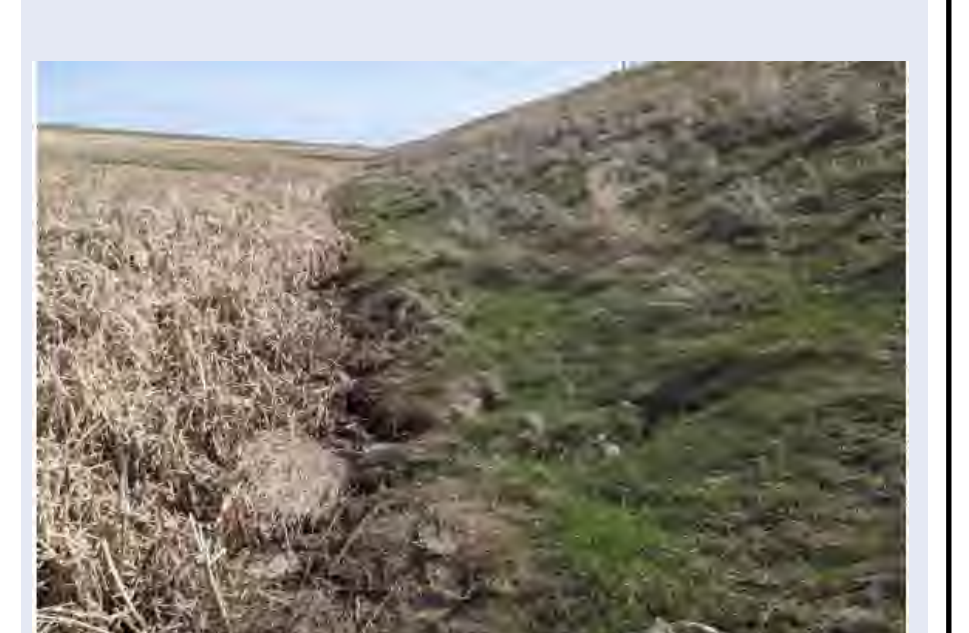
Erosion and movement along Toe
