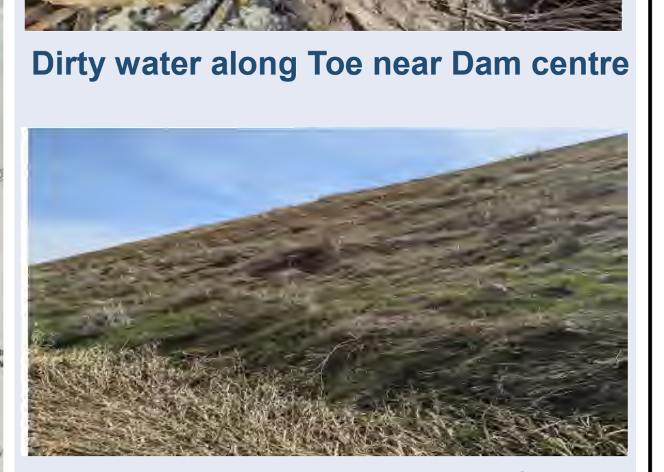
Downstream slope: uneven surface
