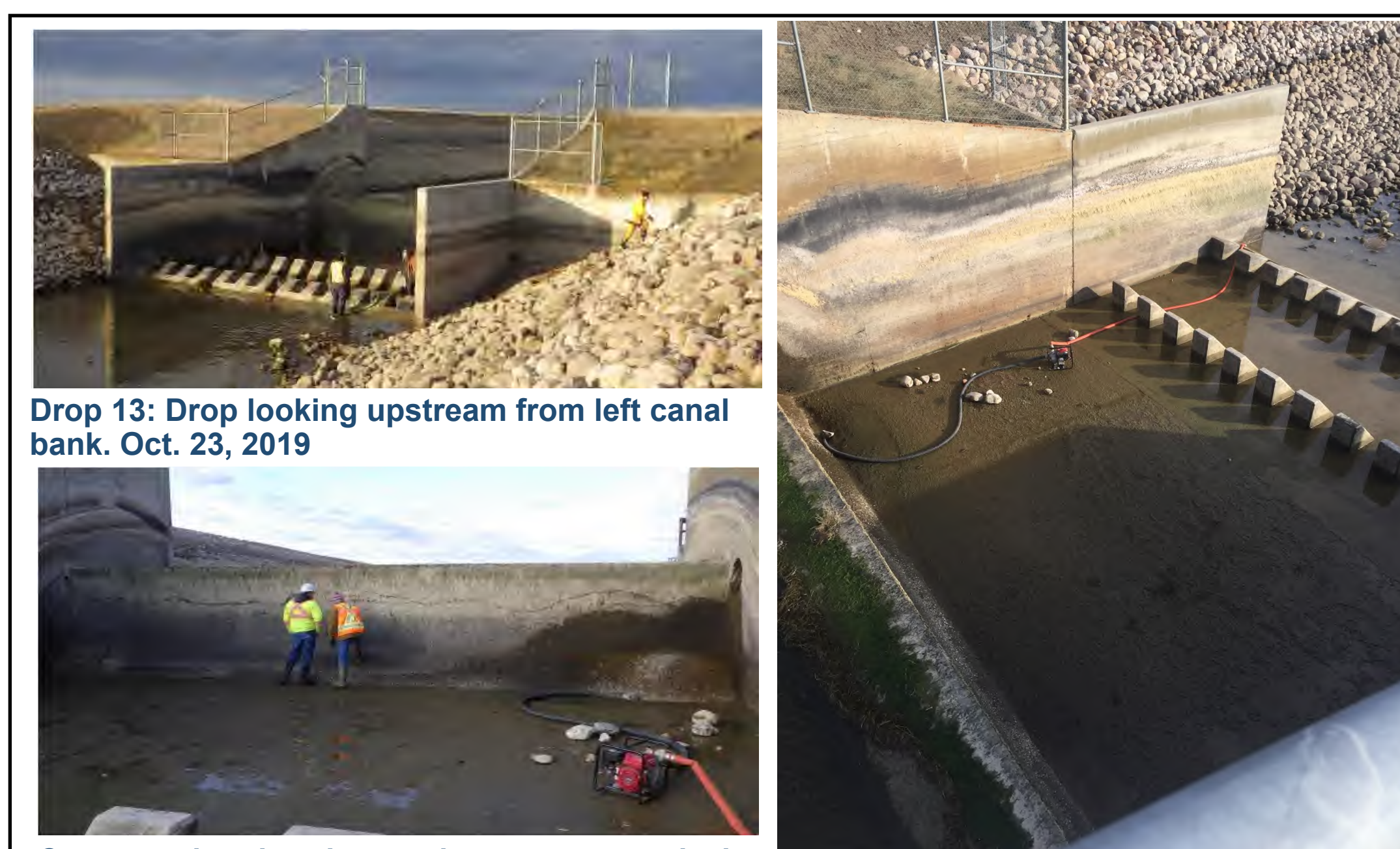
Drop 13: Drop looking upstream from left canal bank. Oct. 23, 2019
