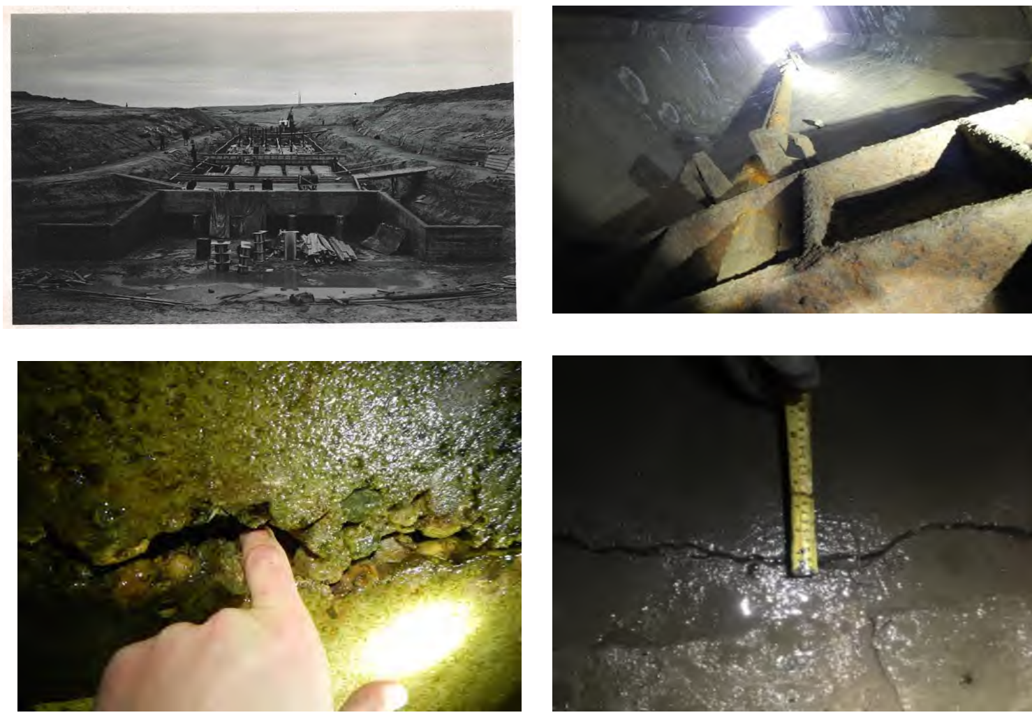
Conduits constructed in 1953 are in "Poor" Condition
