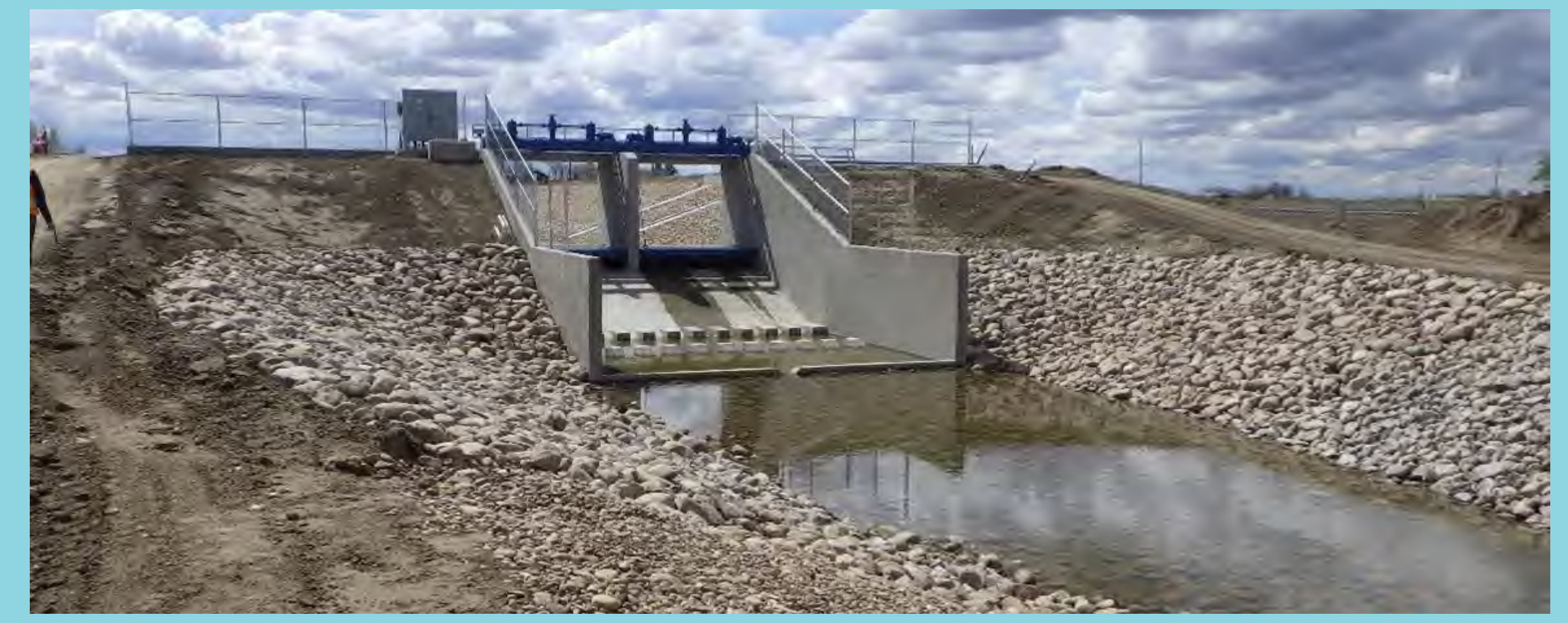
Typical Check Drop Structure Replacement
