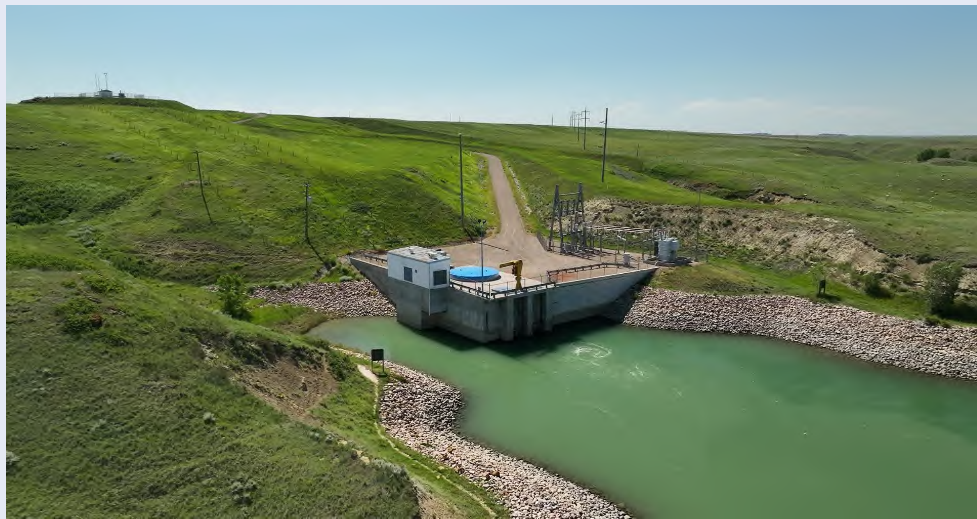
Chin Hydro (11 MW). The was constructed in 1993/1994 and has a vertical Francis turbine and a 40.5 m Head from the upper main canal to Chin reservoir
