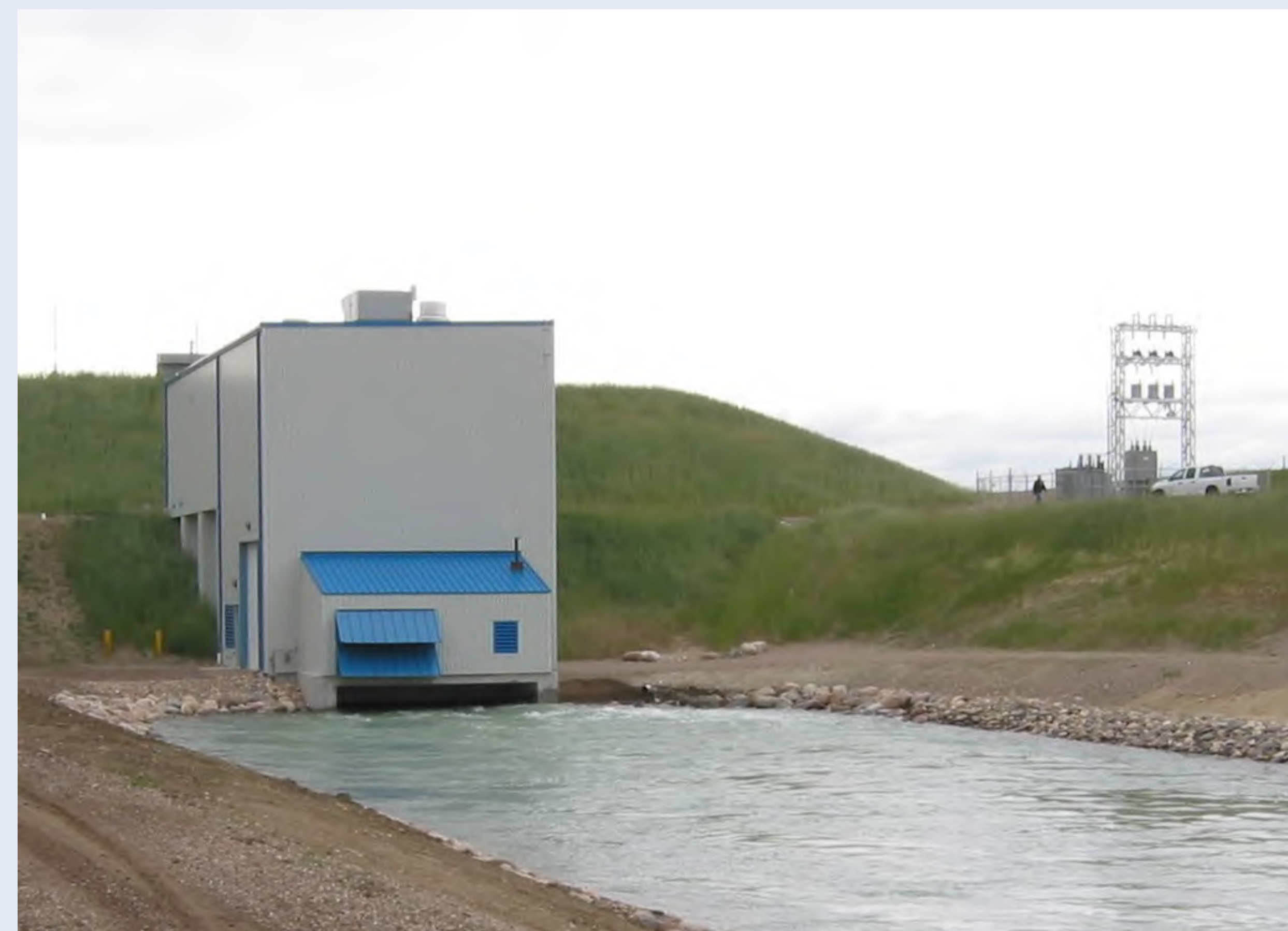
Drops 456 Hydro (7 MW). Located west of Raymond, the site was constructed in 2003/2004 & combines the drop of 3 main canal structures through the penstock.
